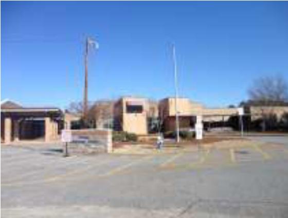
Pickens Elementary School to the west.
